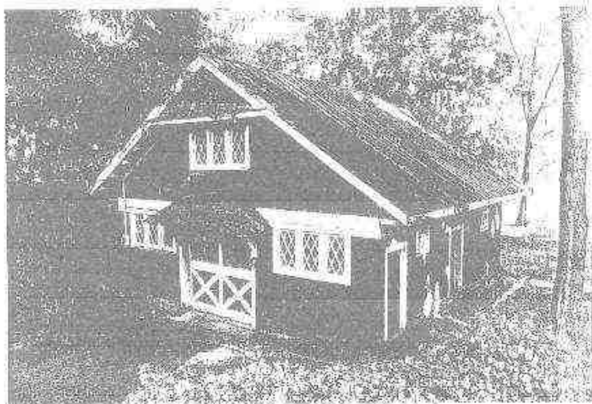
Figure 47. View of the Carriage House from the northwest.
